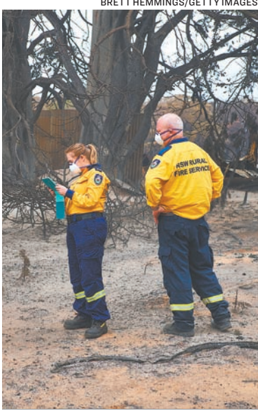
An RFS assessment crew walks through a property recording damage after fire previously tore through the town of Wingello, NSW, on Jan. 6, 2020.
